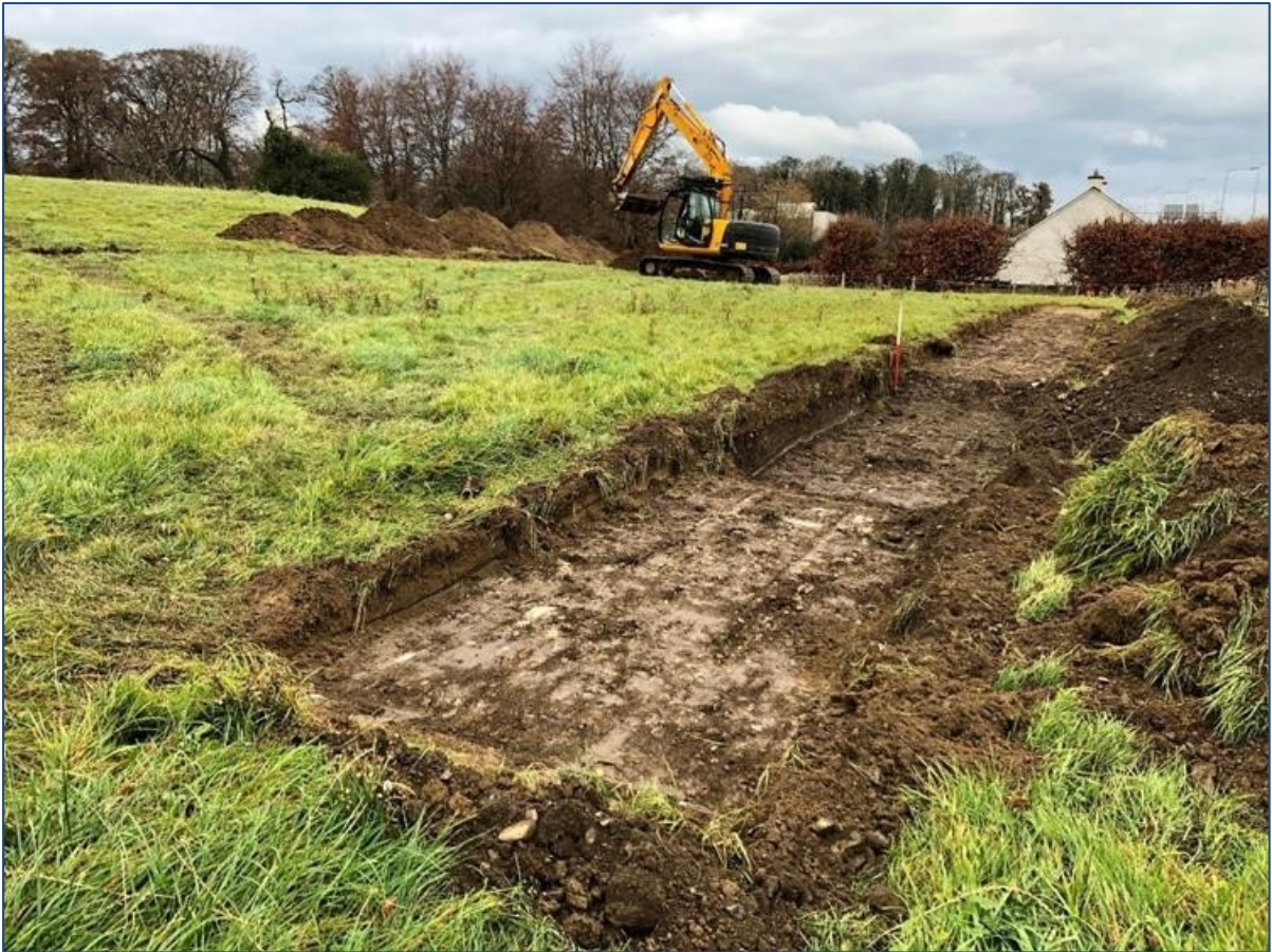
Plate 41: Trench 4.1, with Trench 4.2 in the background facing east-northeast
