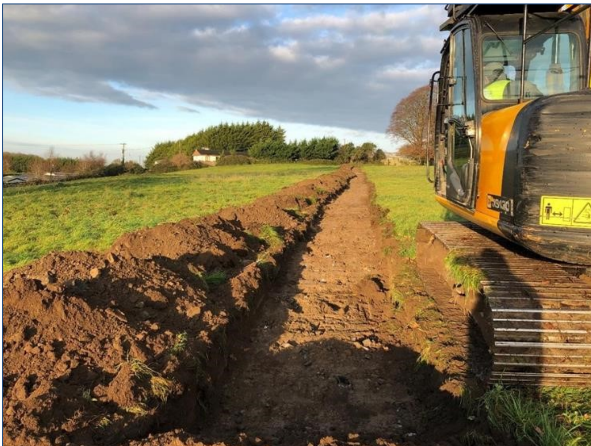
Plate 44: Trench 4.3, facing northwest
