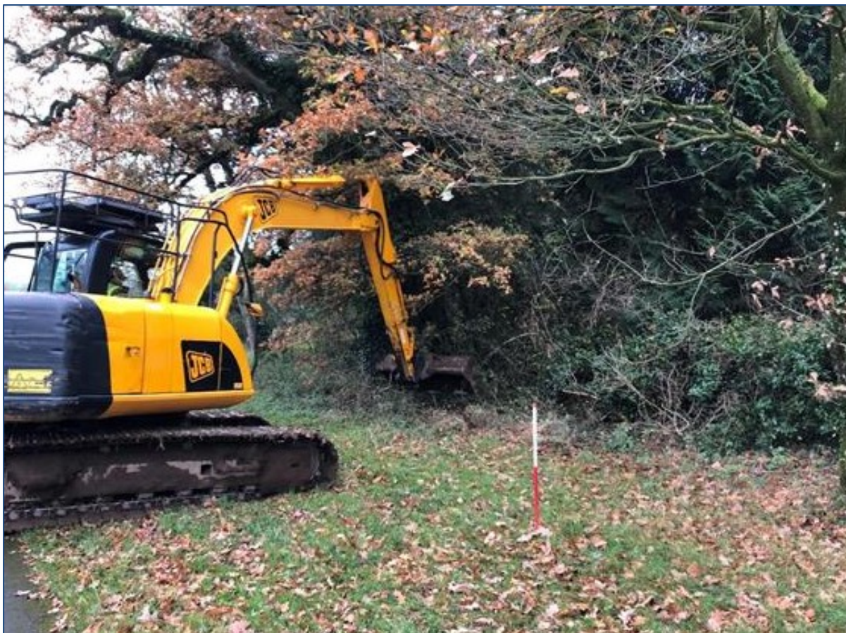
Plate 27: Trench 2.9, breaking ground, facing south
