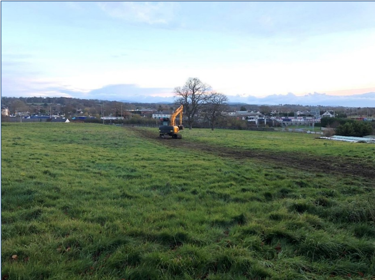
Plate 48: Careful backfilling of Trench 4.3, Field Location 4, in progress
