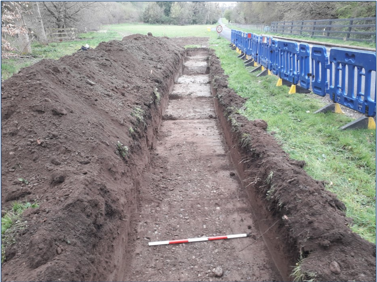
Plate 51: Trench 6.1, looking northwest
