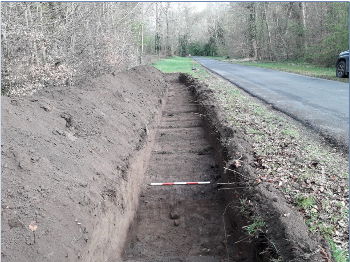
Plate 52: Trench 6.4, looking north-northwest
